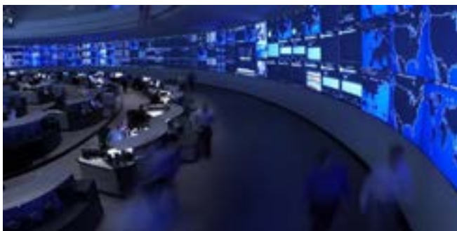
Figure 3 Telecommunications and network operation (Source: http://fortune.com/att-global-network-operations-center/ )
