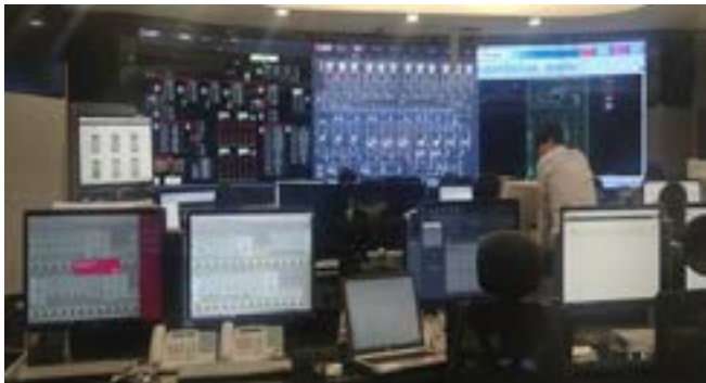
Figure 9 Medium control room
